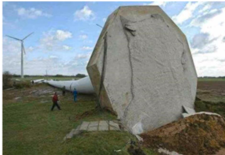
Storm & Tornado, Fallen Wind Turbine
